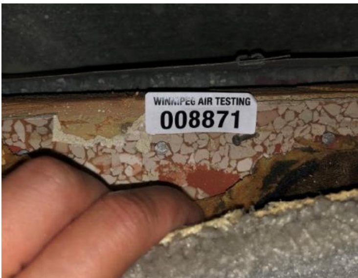
Image of Asbestos Flooring Found under Carpeting
