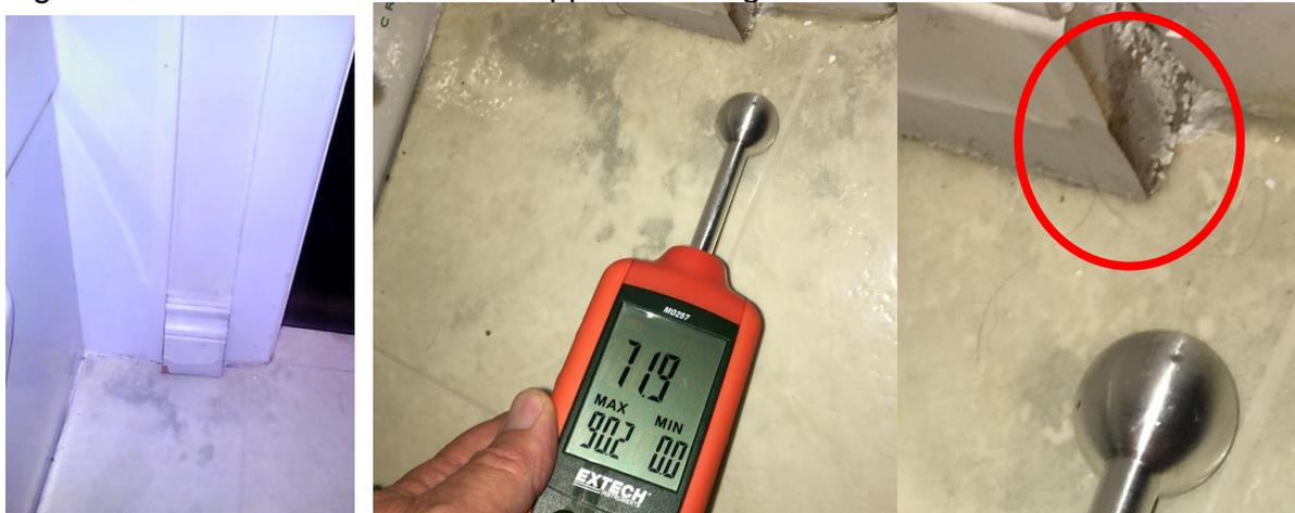
**Left.** Adjacent to the bathtub, visible discolouration of the floor can be seen. **Middle.** A moisture measurement shows high moisture content in the floor (72% moisture content). **Right.** A magnified image shows that the baseboard is visible wet.
