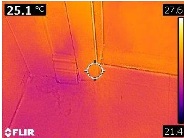
**Above.** Adjacent to the bathtub, visible discolouration of the floor can be seen. The infrared camera shows the floor and the lower part of the wall to be cold due to presence of moisture.
