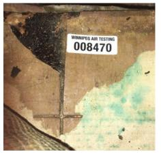
Asbestos containing materials may be obvious. Older walls or floor may have been covered with newer materials. An asbestos audit should consider that some building materials may be hidden under carpeting or behind newer panelling.
